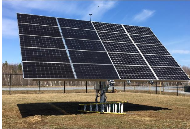
Figure 2-24 – A tracker with 10 monofacial modules (right) and 10 bifacial modules (left).
