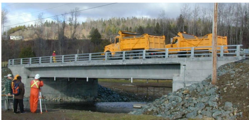
Figura 3: Ponte Wotton Bridge
